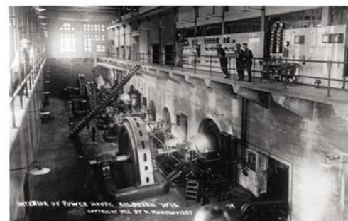
Interior - Turbines (PHS)
